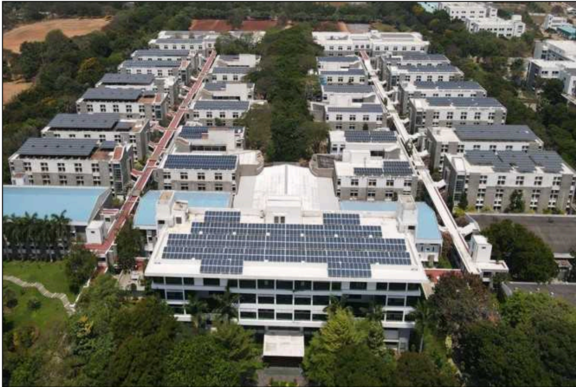
Roof Top Solar Power Plant
