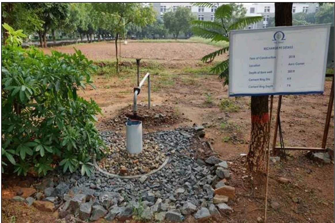
Rain water Recharge Pit
