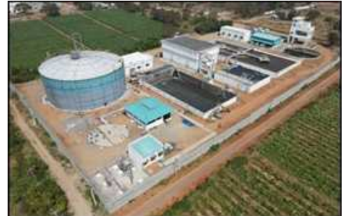
Sewage Treatment Plant (STP)
