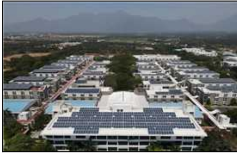
Solar Panel System
