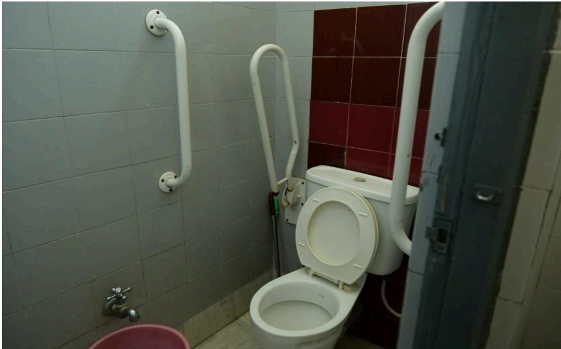
Rest Room with Grab Bars for limited mobility persons
