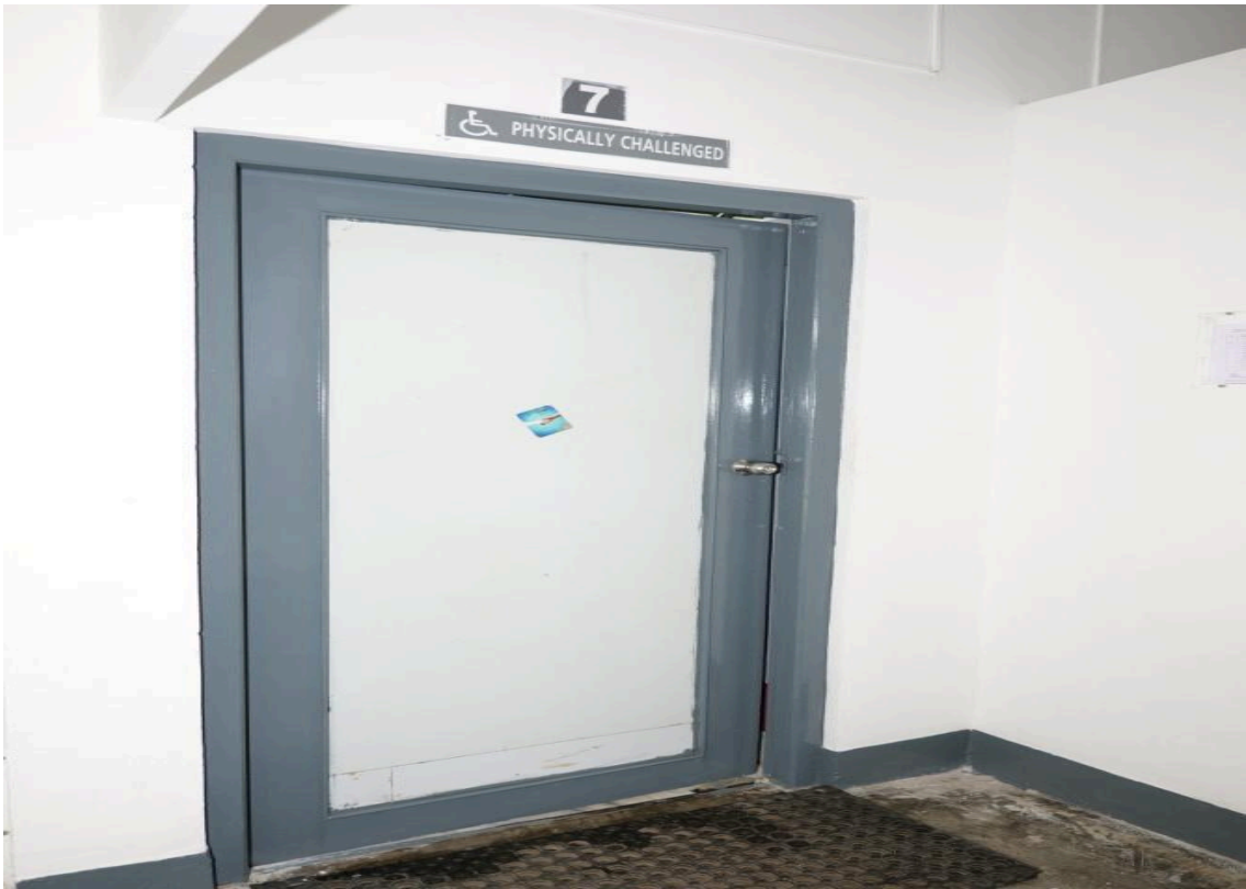
Rest Rooms - Physically Challenge
