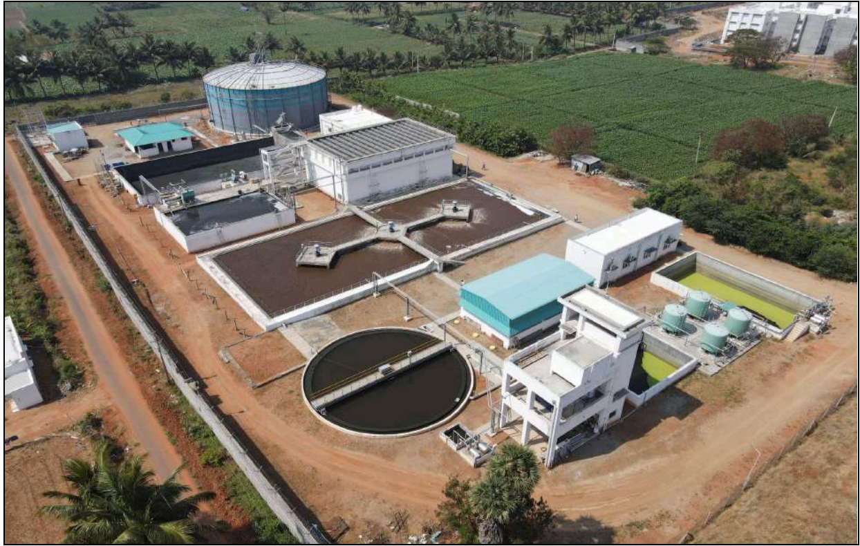
Sewage Treatment Plant (STP)
