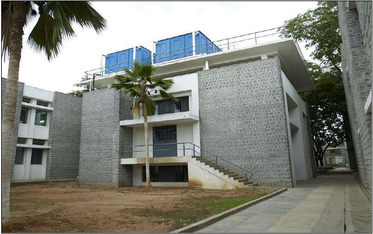
Chiller Plant Facility
