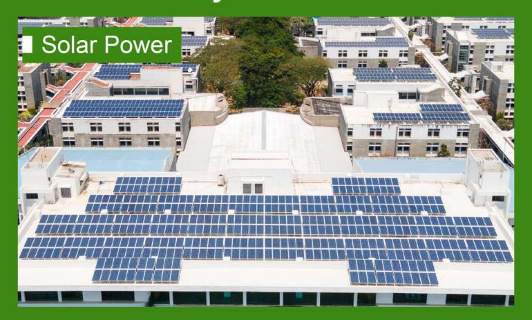
Solar PV system capacity - 1300 kW Battery backup system - 100 kW Local grid tieup system - 900 kW
